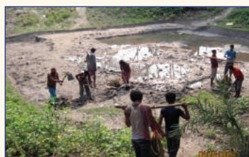
Pond renovation work
