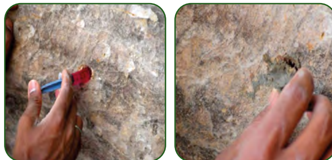
Fig. 7.21: Injecting chemical and seal the hole with mud
