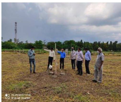
Site selection for installation of Agro Automatic Weather Station
