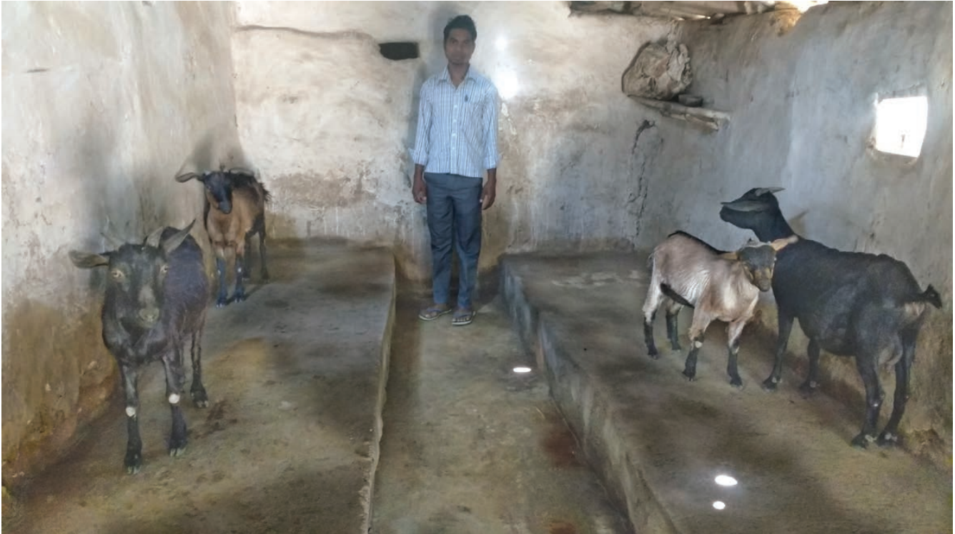
Photo 28. Raised cement floor for goat keeping at Burhakocha, Ranchi, Jharkhand
