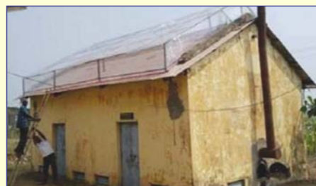
Curing barn with polycarbonate roof top
