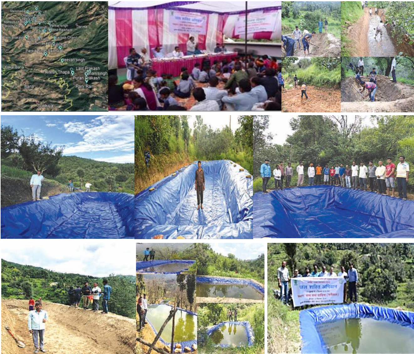
Low cost polytanks for enhancing water productivity at Darima village, Nainital under Jal Shakti Abhiyan Programme
