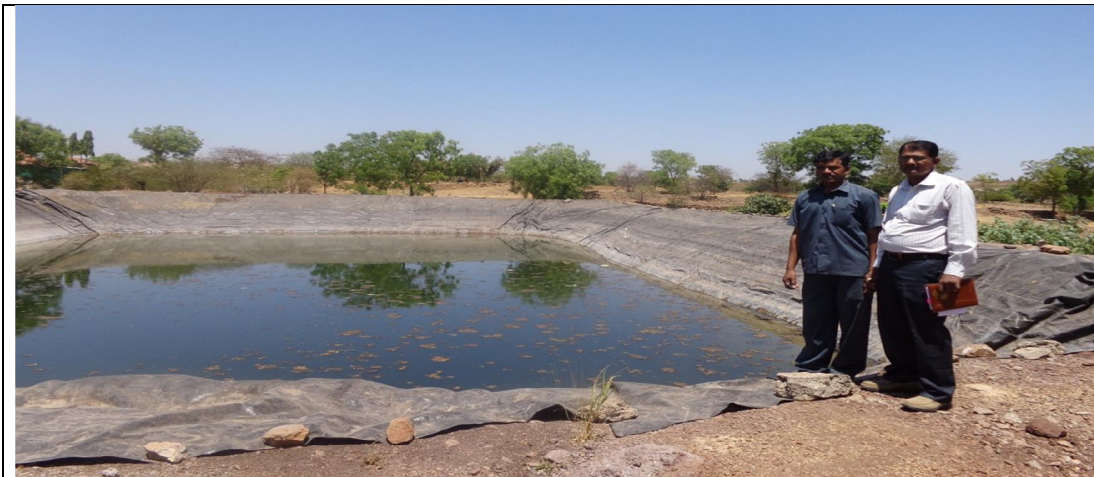
Farm pond constructed under the scheme Farm Pond on Demand implemented by Govt. of Maharashtra
