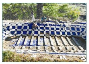
cm/  $50 \times 20 \times 6$  cm. The tank was constructed at the experimental farm and farmers' fields. Since year 2012, 23 tanks have been constructed at farmers' fields which are functional till-date. The tank is durable with an expected lifespan of 45 years.
