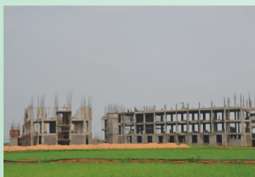
Admin building (side view)
