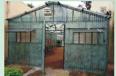
Insect Screening Facility
