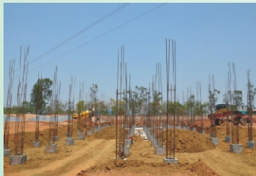
Initial stage of building
