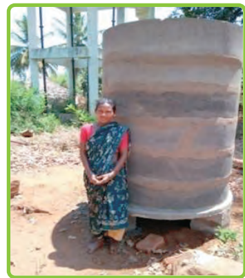
Improved concrete grain storage structures introduced
