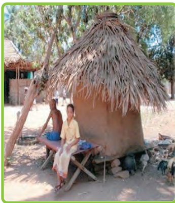
Existing grain storage structures (Mud plastered bamboo covered with palmyrah)
