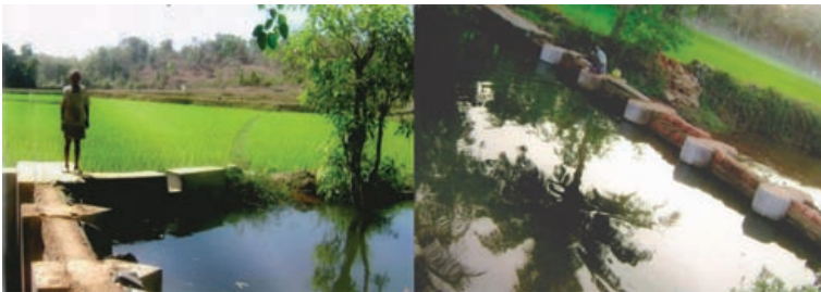
Figure 2: Vented dam- Watershed development Department Uttarakannada Taluk: Siddapur
