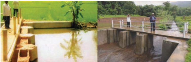
Figure 4. Foot bridge over the vented dam
