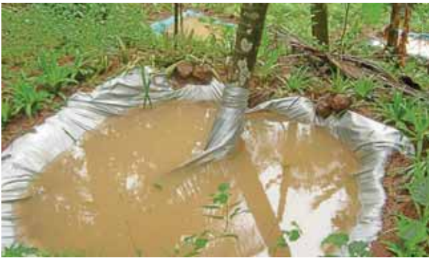
Fig. 65. Water conservation structures using plastic sheet
