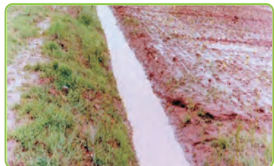
Safe disposal of excess water
