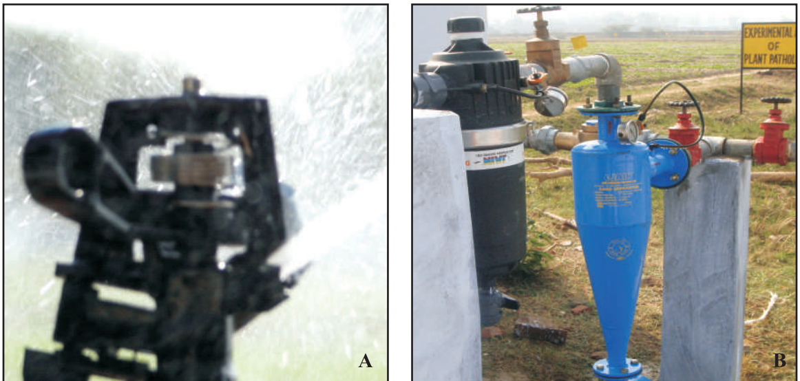
Fig. 6. A. Part circle micro-sprinkler head in action, B. fertigation system with hydrocyclone and disc filters
