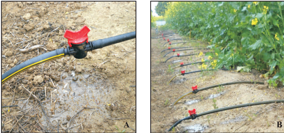
Fig 7. A. Drip lateral alongwith regulating valve, B. lateral in between mustard rows
