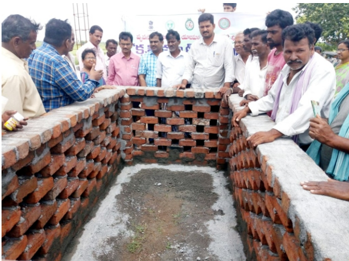
Nadep compost pit at Khammam
