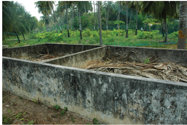
Vermicomposting in tanks at Minicoy
