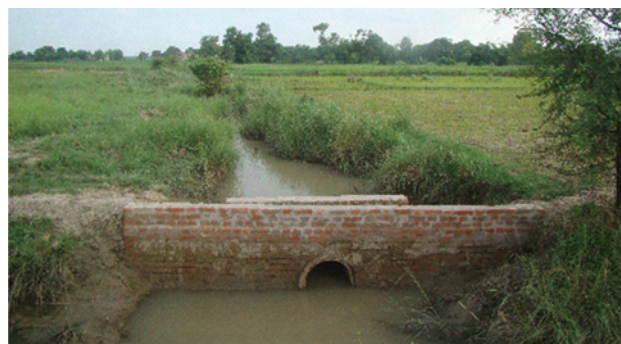
After construction of retention wall-cum-drainage (Dimension: 15' X 5' X 1.25')
