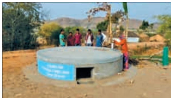
Rainwater harvesting tanks of 21,000 liters capacity at Bernia watershed (Dungarpur)
